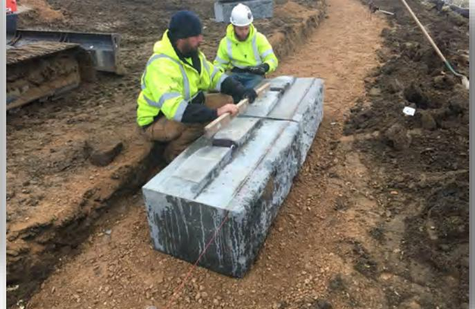
Walls should generally be built starting at the lowest elevation along the wall. However, if there are corners and/or abutting structures along the wall profile, these locations may be better places to start construction.
