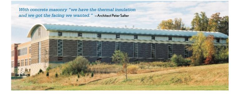
building's wall would show an exterior face shell 1.5 inches (38 mm) thick, a oneinch (25.4 mm) cavity for water drainage, two inches (50.8 mm) of rigid insulation for thermal performance and three inches of grout. Builders installed cabling and conduits in the cavity between the insulation panel and the 1.5-inch-thick interior face shell, then filled the remaining space with 3,000 psi concrete grout.
