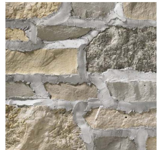
OVERGROUT JOINT
